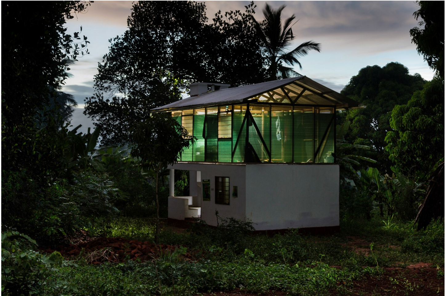
Fig 4. An example of novel-design, double-story building in Magoda, Tanzania. Indoor illumination illustrates the light- and air-permeable character of shade net cladding (photo by Konstantin Ikonomidis).
